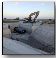
Installation of new HDPE pipe into the existing piping along the E65 system north of Bertrand
