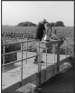
Raising gates — Irrigation Service Specialist Keith Jauken uses a tool to raise a canal gate to allow a higher flow of water to enter his canal during irrigation season.
