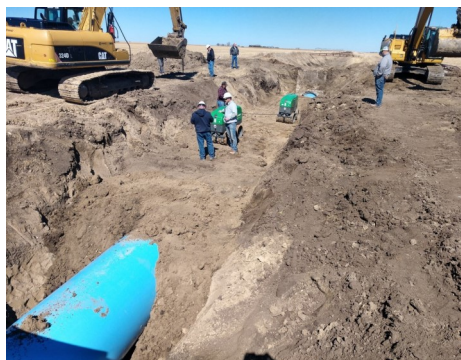
Central employees work to install a new pipe and conduit for a road crossing near Loomis.
