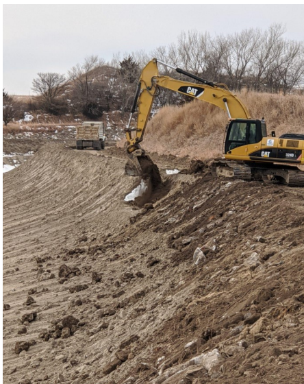
A Central equipment operator uses an excavator to lay rock along the side of the Phelps Canal.
