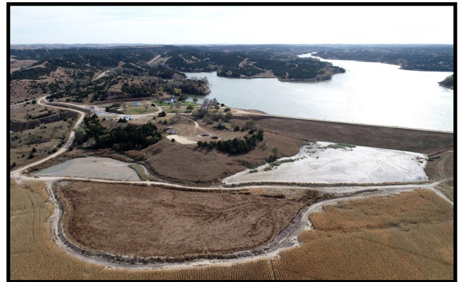
Drone photo taken by Central staff showing Jeffrey Reservoir and the silting ponds used during dredging projects over the past years. These settling ponds were made possible through a collaborative effort between the land owner, tenant and the District.
