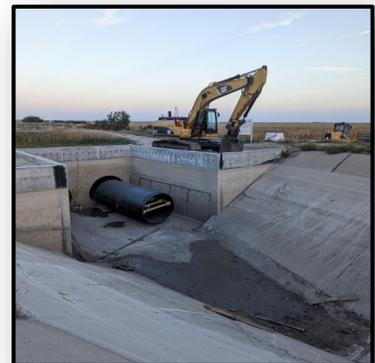
*Installation of new HDPE pipe into the existing piping along the E65 system north of Bertrand*
