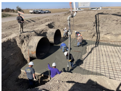
Central employees pouring concrete along the E65 system
