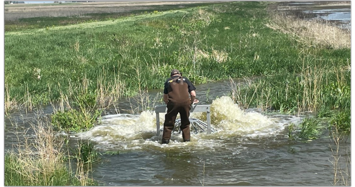
Irrigation Service Specialist Keith Jauken opens the gates to deliver water into Funk Lagoon. This recharge occurs with excess flows within the basin
