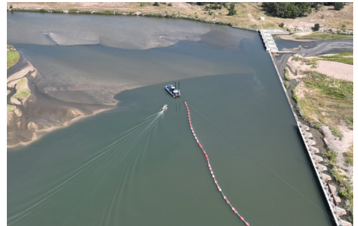
Drone footage of the new dredge in use at the Supply Canal dam that shows the sediment being removed
